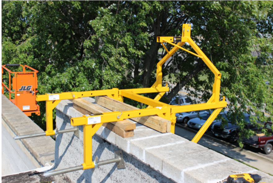
Window Outrigger Components
