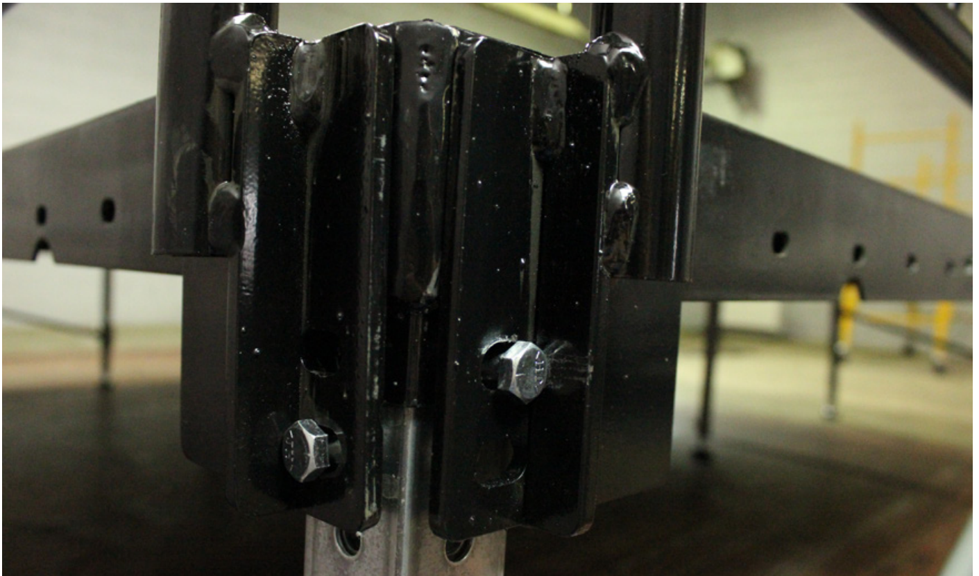
Closeup of guardrail attached to stage corner.
