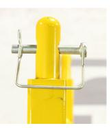
clearly require that the ladder sections be physically attached one to the other. Uplift could occur by simply climbing the scaffold if the ladder sections are not pinned together.
