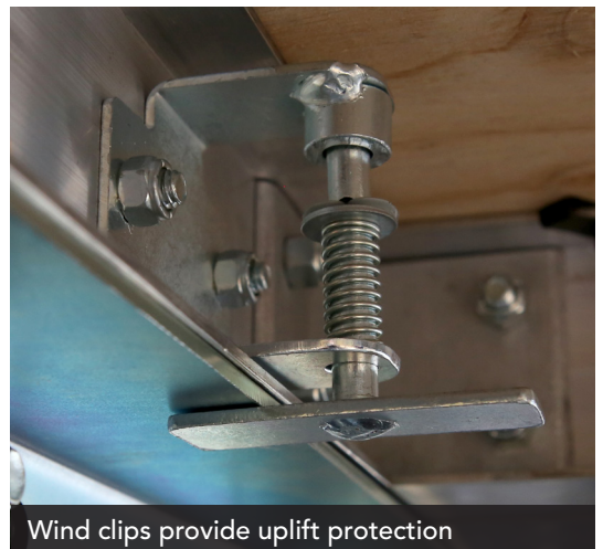
Beam support pin
